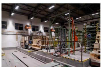
The workplaces of the presses were illuminated by individually switched luminaires. DALI control allows to set different levels of illumination for each activity. The use of energy saving and temperature resistant LED luminaires combined with **DALI control with daylight and motion sensors** give a superior **76% operating cost savings** to the customer **with a 40% increase of illumination level**.
